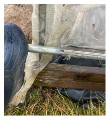
Figure 12.9 Tapping curtain poles down with one's foot.
