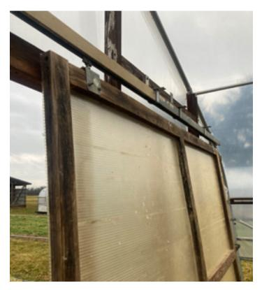
Figure 12.6 Sliding door hardware.
