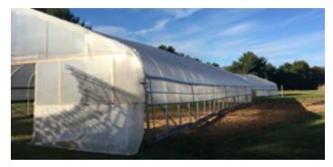
**Figure 12.4** Windstorm-shifted tunnel. Windstorms moved tunnels when anchors had not been fully installed. Note the structure has been picked up and moved diagonally in the plot.
