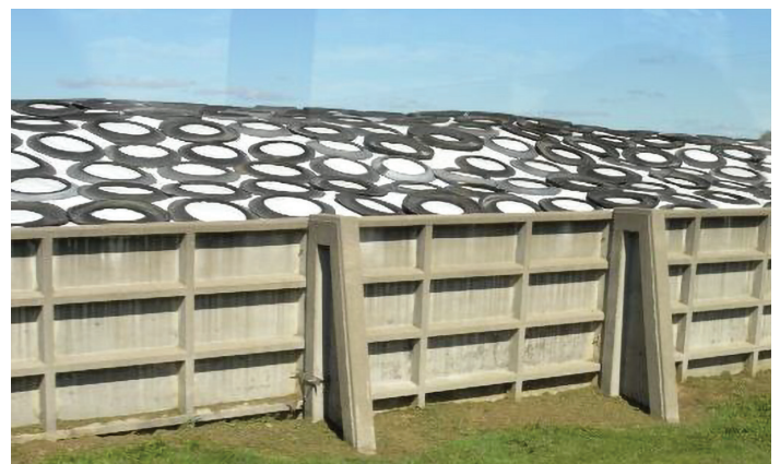
Figure 7. Bunker silo with plastic covering the top weighted down with tire walls. Photo: Donna Amaral-Phillips.
