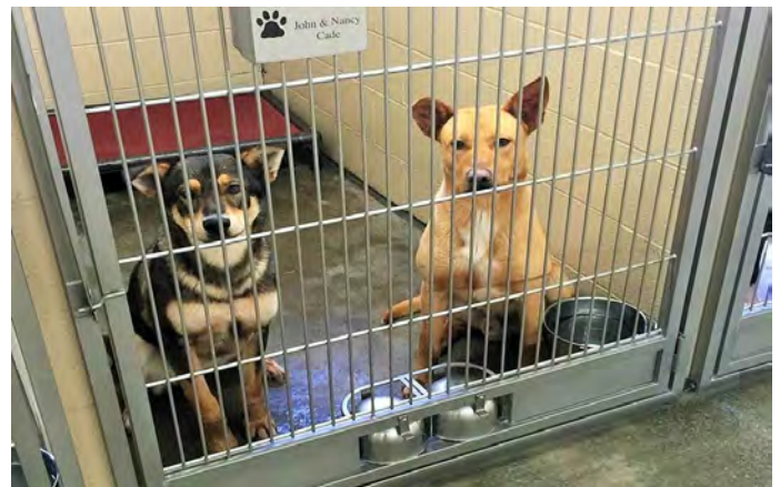
Dog kennels built of impervious materials that can be easily cleaned and disinfected
