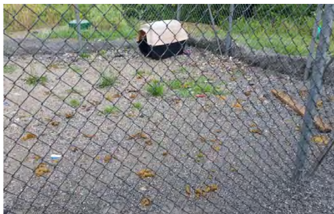
Example of dog pen with gravel floor that cannot be disinfected and not adequately cleaned
