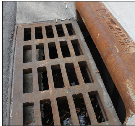
Figure 1. Trash can enter the storm sewer systems through curb inlets, located in parking lots and along roads.
