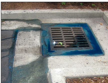
Figure 1. As runoff flows over the land to waterways, it can pick up pollutants such as sediment, nutrients, and pathogens.
