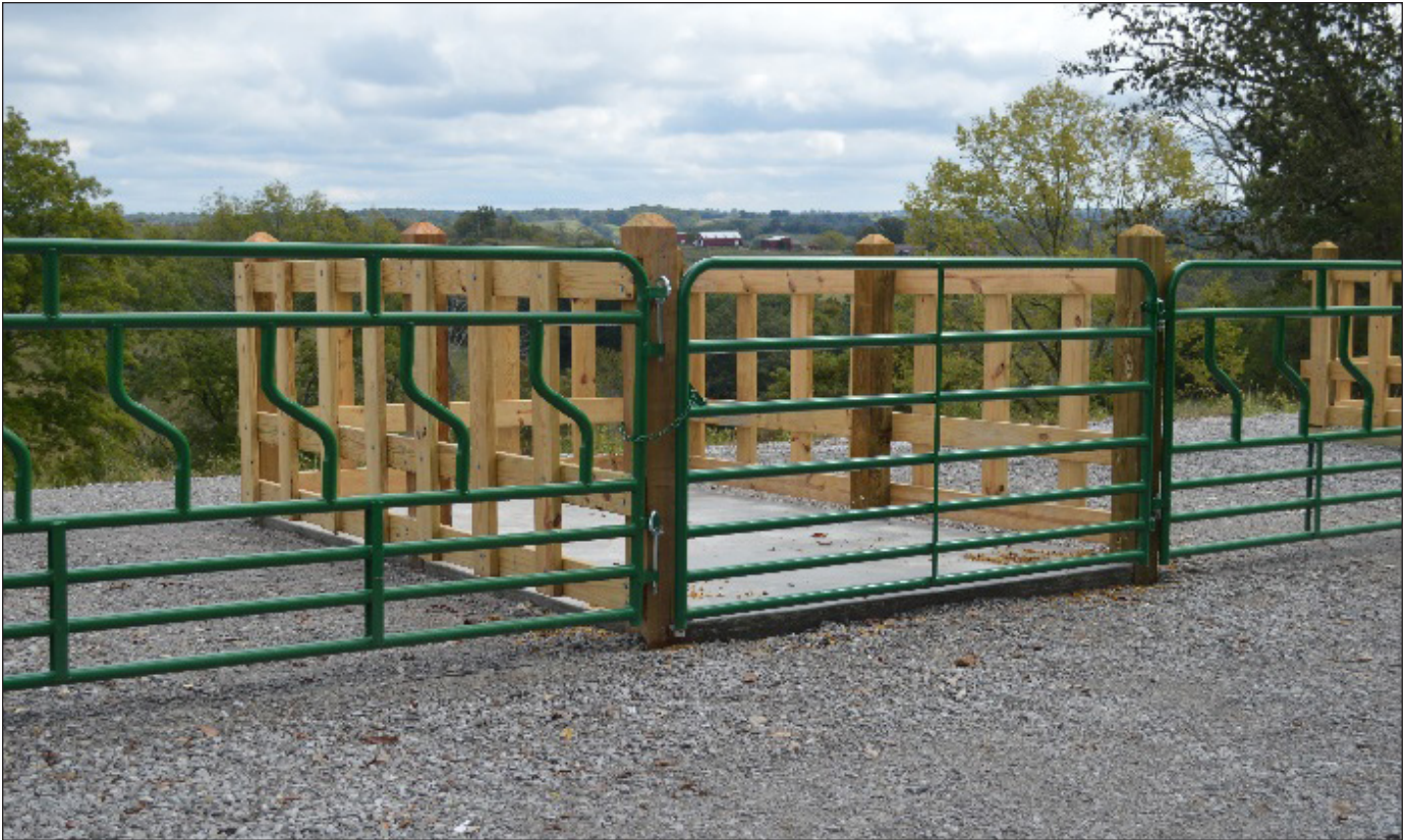
Option 3. Uncovered structure with wood panels and geotextile fabric, grid, and gravel pad surrounding.
