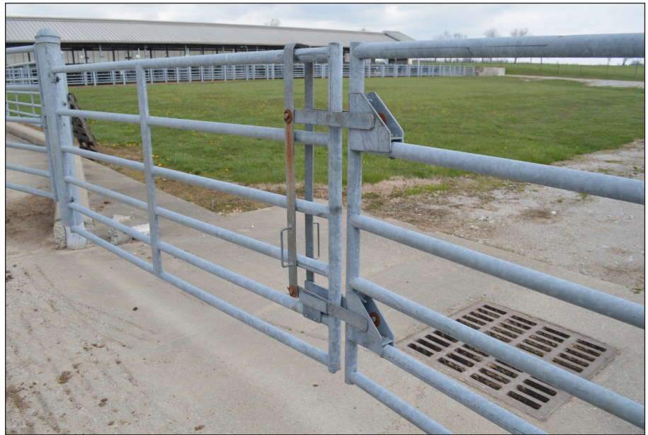
Figure 3. This heavy-duty gate utilizes a reinforced drop-over catch mechanism that ensures closure of the gateway and provides peace of mind to the producer. Photo by Steve Higgins
