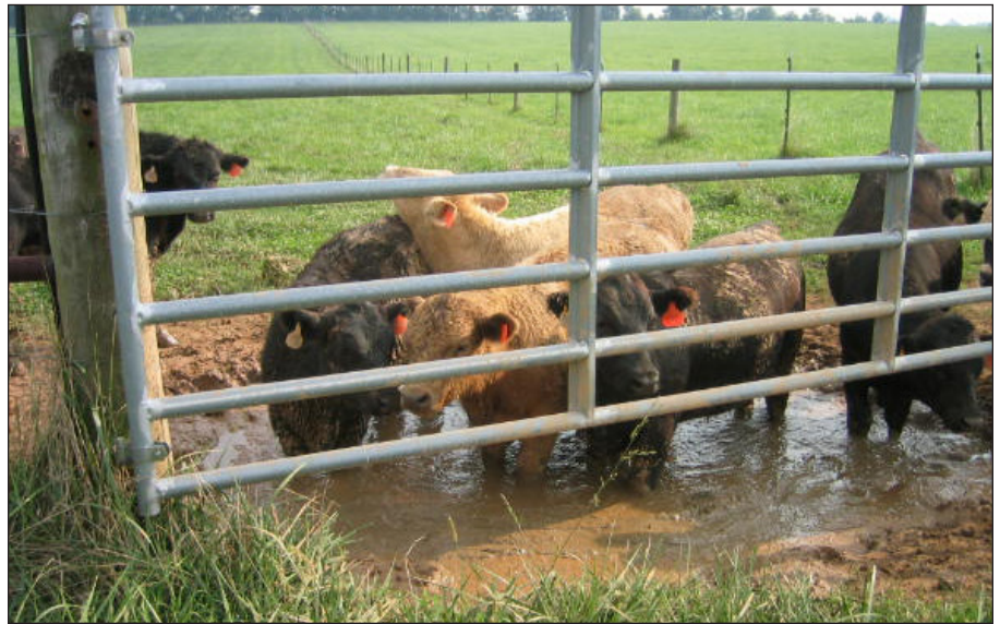
Figure 5. An extreme example of the damage that can occur when a heavy traffic pad is not installed in a gateway. Photo by Glenn Aiken
