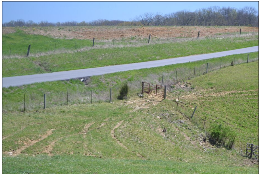
Figure 4. Drainage water should not run through or across a gateway. Photo by Lee Moser
