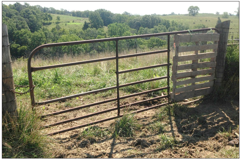
Figure 7. The need for gate repair is inevitable. Repairs should maintain the original integrity of the gate and be able to restrict the movement of livestock. If a gate is no longer resistant to livestock pressure then it is time to replace the gate. Photo by Dan Miller
