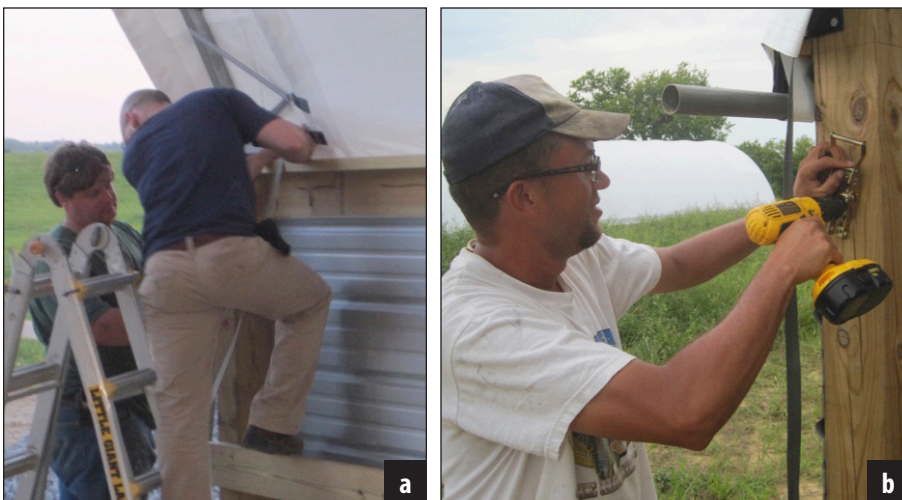
Figure 24. Finalizing the lacing on the end and attaching a small ratchet to cinch in the end of the tarp.
