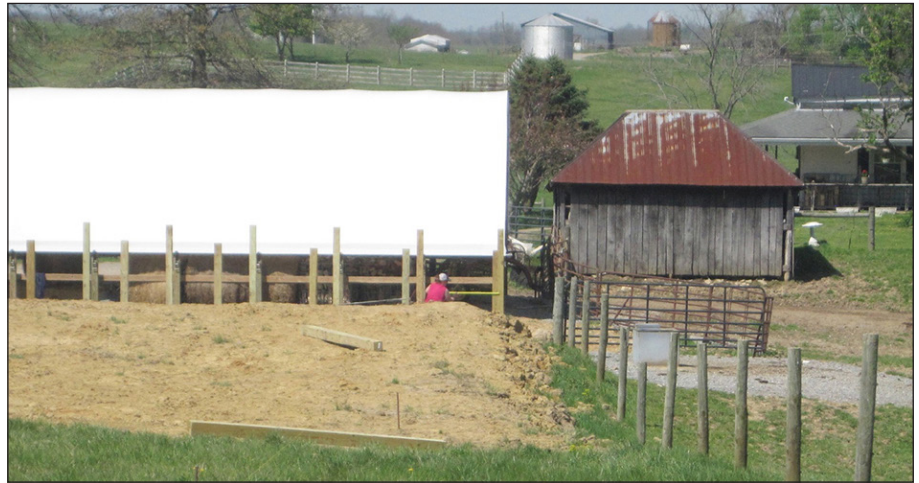
Figure 1. Hoop barns require a level spot with decent drainage.
