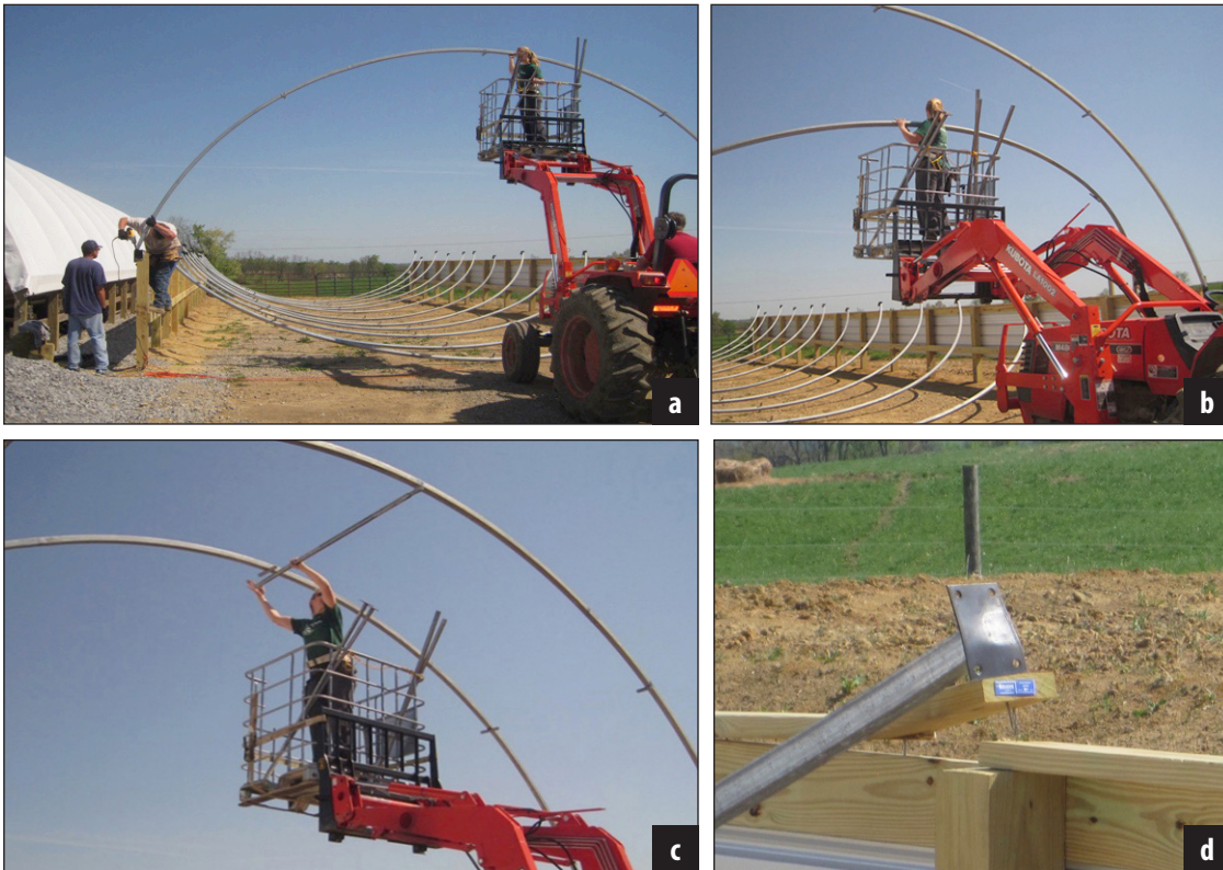
Figure 14. Lifting the ribs and attaching them to the knee walls.
