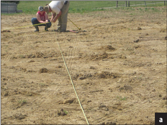
Figure 3. Identifying the hoop barn's third and fourth corners and representation of the dimensions that would be measured with the tape measures when identifying locations for corner posts.
