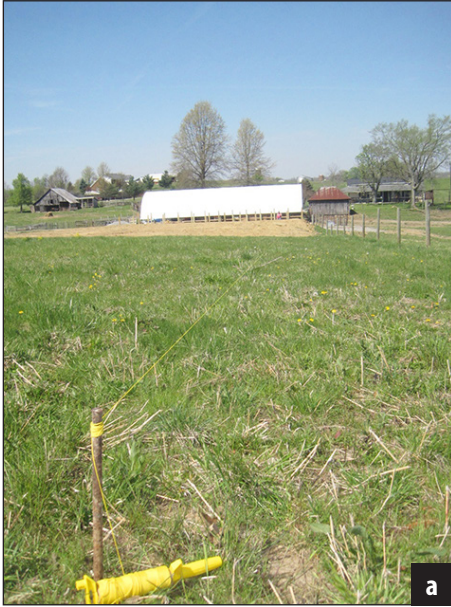
Figure 2. String lines for the hoop barn.
