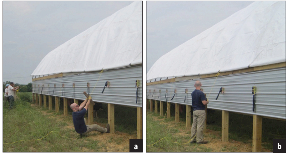
Figure 20. Leveling out the tarp along each sidewall to ensure ratchets will work.
