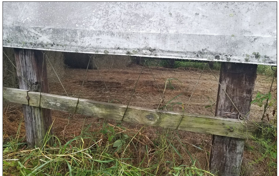
Figure 22. Lacing to hold the tarp along the sidewall.
