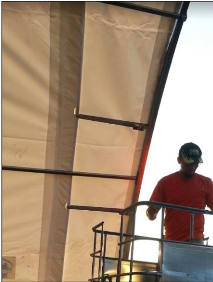
Figure 25. Tarp tightened using ratchets rather than lacing for the end.
