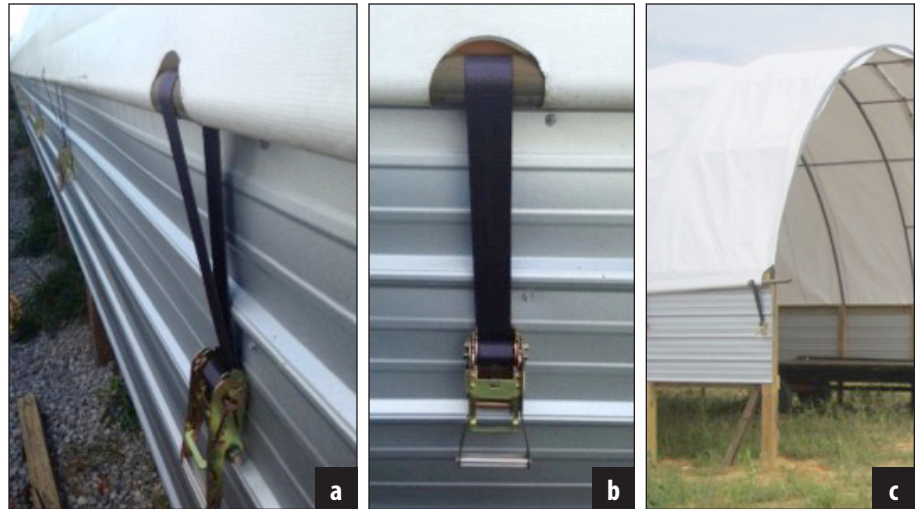
Figure 21. Ratchets to hold the tarp along the sidewall.
