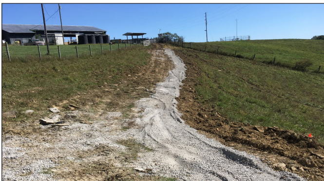
Figure 6. A completed trail leads to a water source located on a hill with 30-percent slopes.
