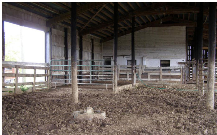
Figure 9. Surfaces for livestock should be created to provide support, drainage, and comfort, unlike this clay-spiced floor previously used in Eden Shale's old dairy barn.
