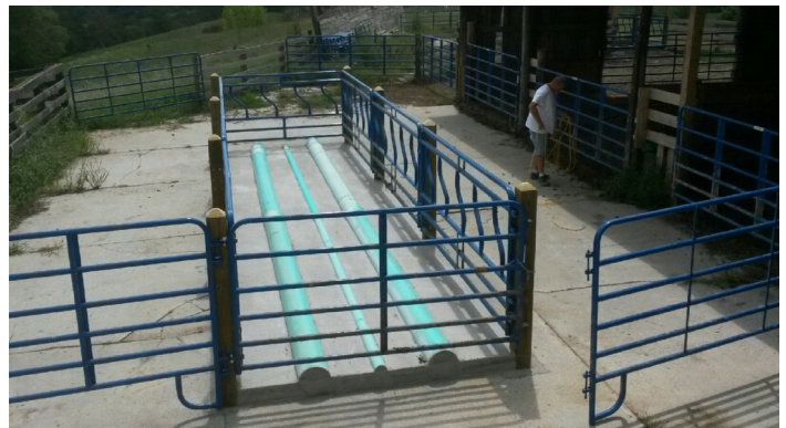
Figure 8. A new hay feeder that provides linear feeding space serves three fields plus two pens inside the redesigned barn. Gates in the foreground allow for manure cleanout, while the gates in the back feed into the pastures and lane.
