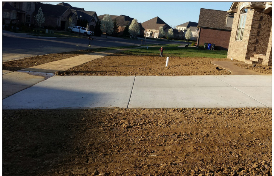
Figure 3. Soil prior to planting seed, sod, sprigs, or plugs should be firm and free of any debris.
