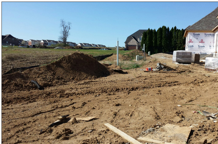
Figure 1. Topsoil stockpiled on the edge of the lot awaiting construction completion. This pile is likely not large enough to provide 4-6 inches of topsoil over the entire yard.
