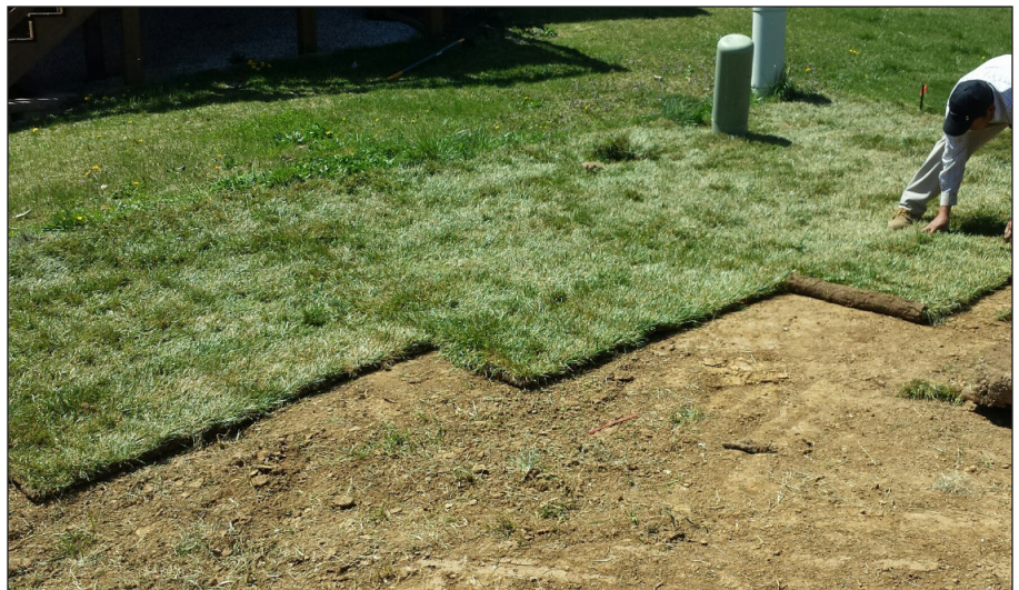
Figure 7. Staggering sod rows minimizes seams and slows water movement down slopes. Laying sod results in a uniform weed free lawn and can be established at almost any time of year.
