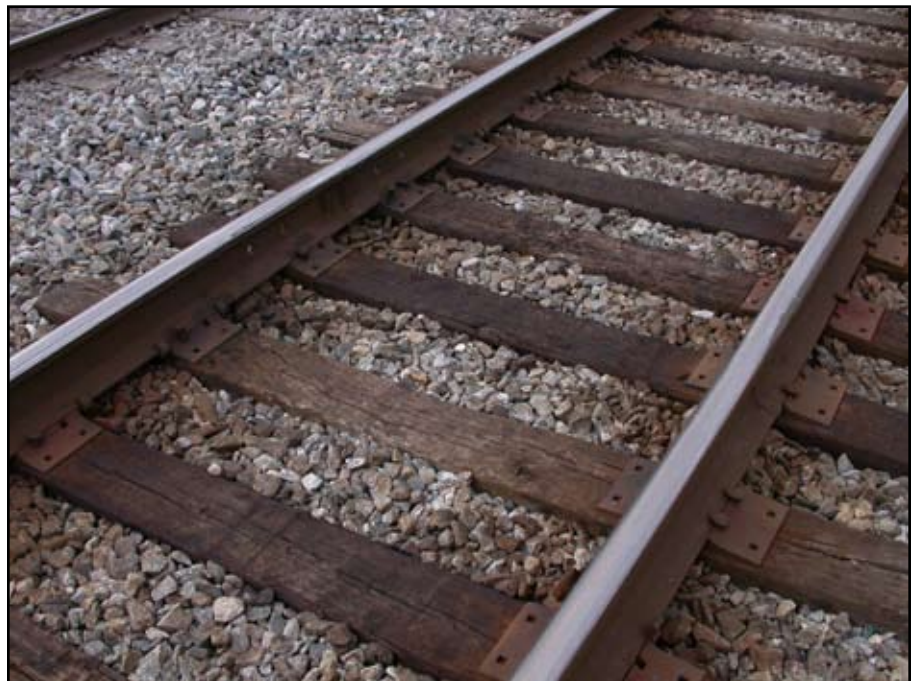
Figure 10. A section of railroad track showing tie plates and spikes.
