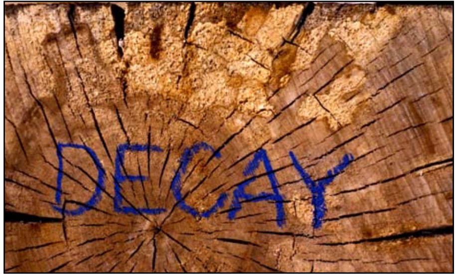
Figure 18. Decay in an air-dried cross-tie.
