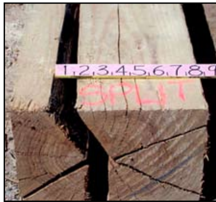
Figure 29. This tie has a split that is over one inch wide, and it's not salvageable.
