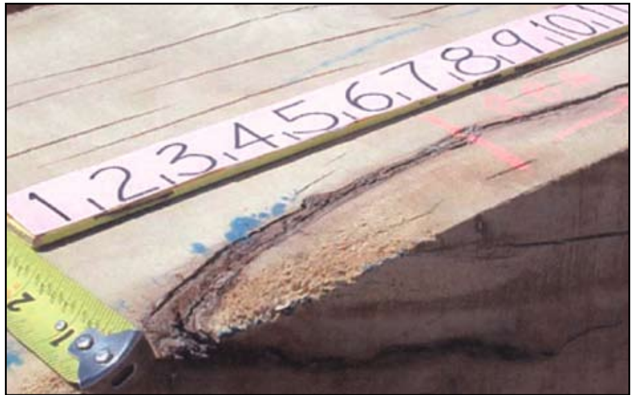
Figure 31. This bark seam is greater than 2” deep, and it’s also longer than 10”. (Look how the bark seam extends from the face and down the side.) It fails to meet the minimum tie specifications.
