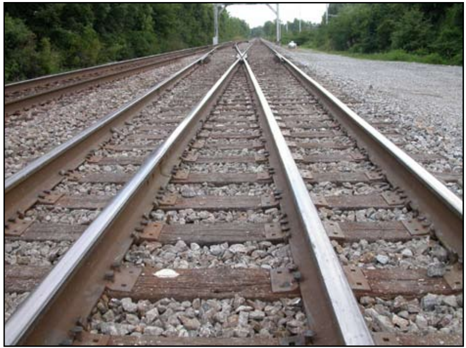
Figure 11. The use of switch ties, where two sections of track are joined by one long wooden tie.
