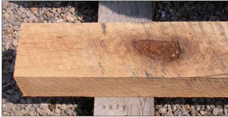
Figure 8. A large rotten knot caused this tie to be culled.
