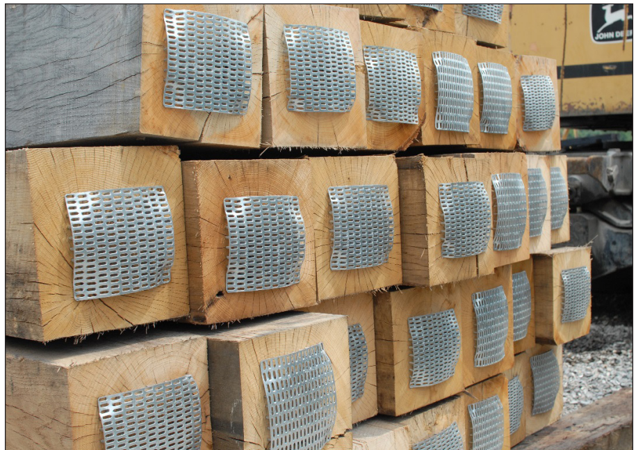
Figure 5. This is an example of crossties with gang nail plates. In this photograph, the plates have been tacked on and they are awaiting hydraulic pressure to seat them to their full depth. If these ends weren't all squarely cut, the nail plates wouldn't seat properly.
