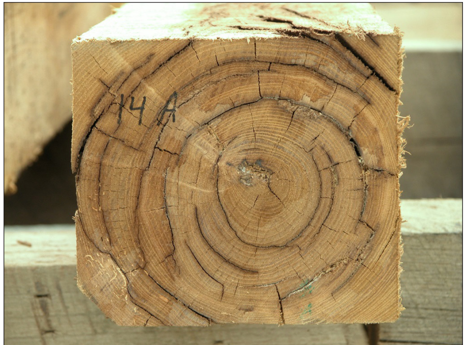
Figure 19. This is an example of really bad shake in a black locust tie.
