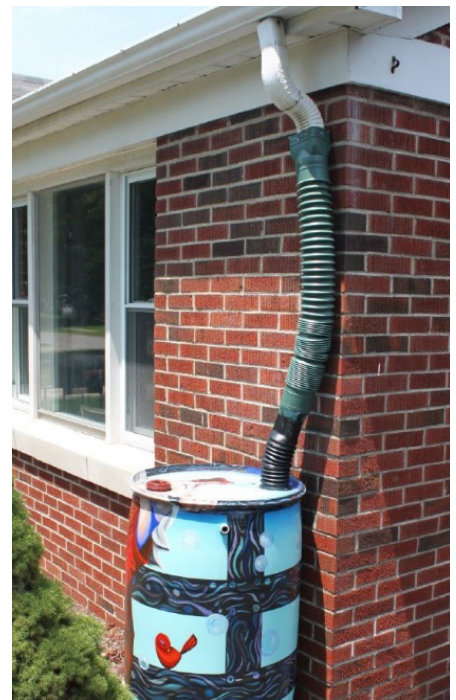
Figure 2. Rainwater harvesting with a rain barrel is a simple stormwater management practice that homeowners can install.
