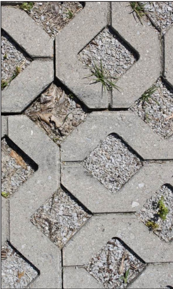
Figure 7. Concrete grid pavers contain spaces that allow stormwater to infiltrate between the pavers. Spaces can be filled with small aggregates (left) or soil and grass (right).
