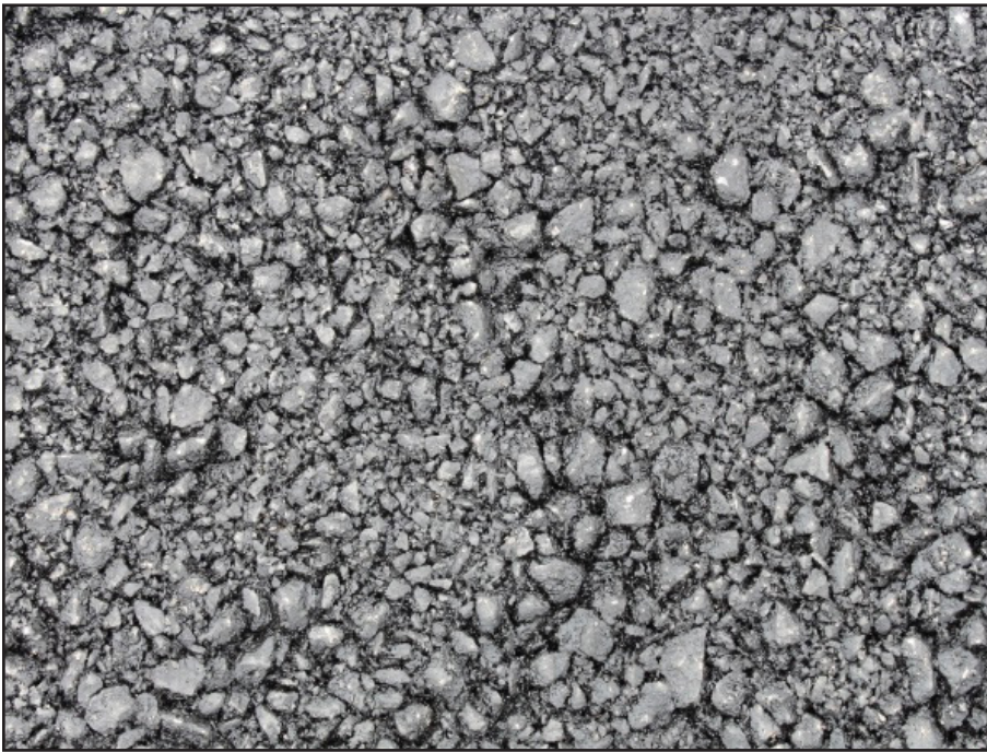
Figure 6. Porous asphalt can be used in low-volume, low-speed vehicular traffic applications.
