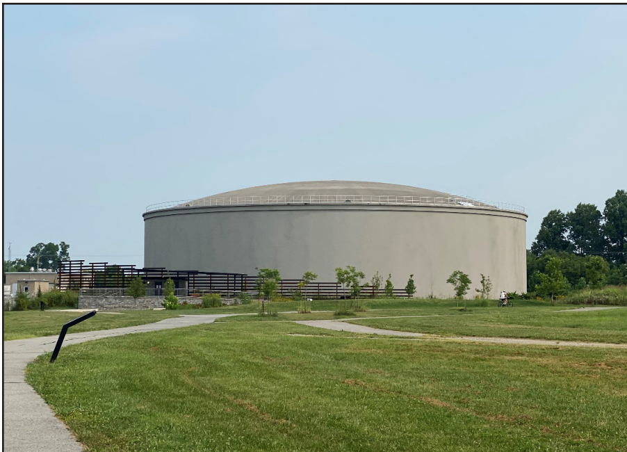
Figure 4. A wet-weather storage tank designed to handle excess sanitary sewer load during high-flow events.
