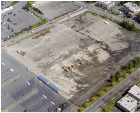
Figure 10. Before, during (below), and after (far right) construction of the Thoraton Creek water quality channel. SVR Design Company 2009
