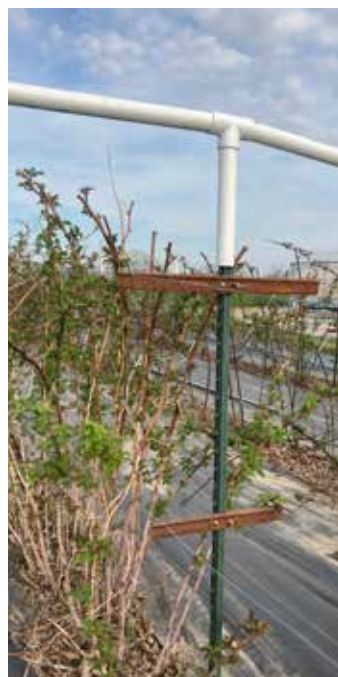
Berry trellis component is made of a metal T-post with two crosspieces and a PVC tee at the top to lift the net above the plants.
