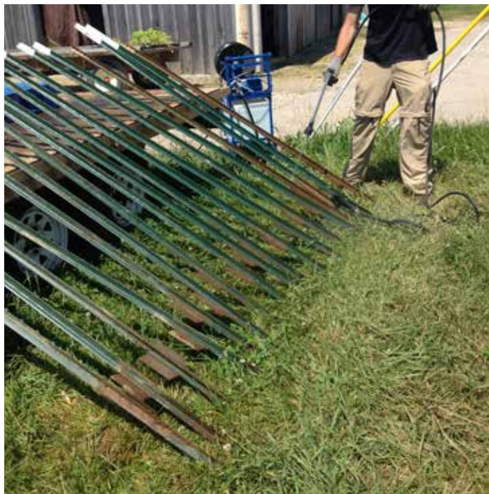
Metal T-posts being sanitized before installation.
