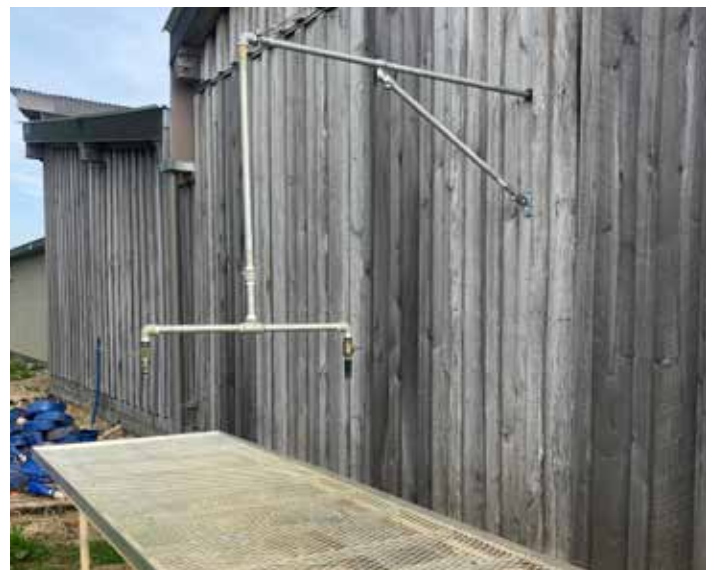
Figure 11.7 Bunched washing station.
