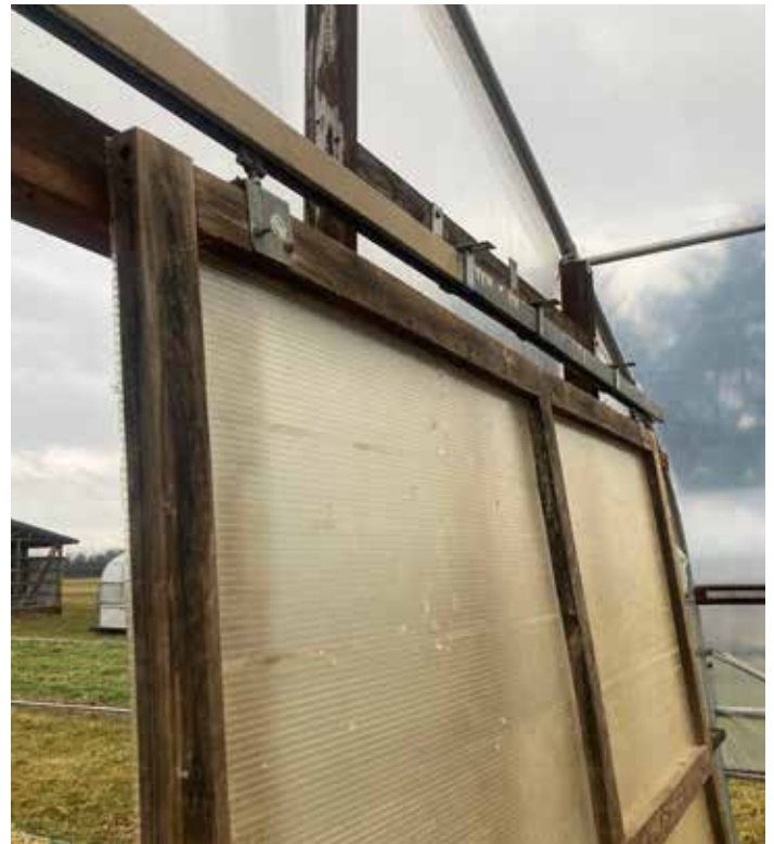
Figure 12.6 Sliding door hardware.
