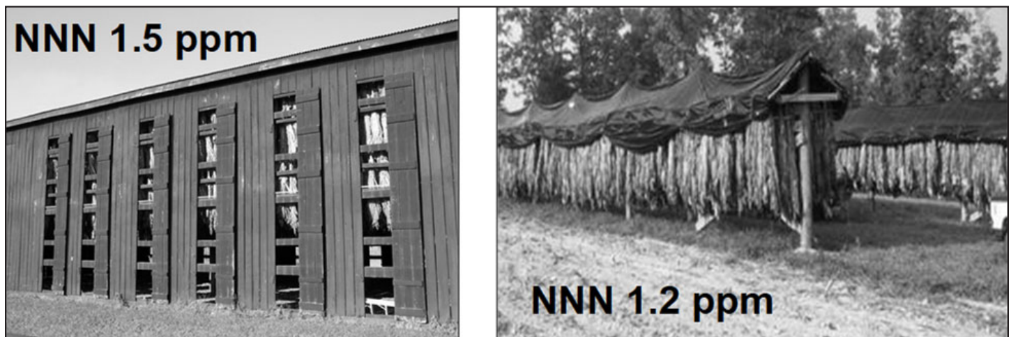
Figure 9. NNN (ppm) in a conventional barn (left) and outdoor curing structure (right).
