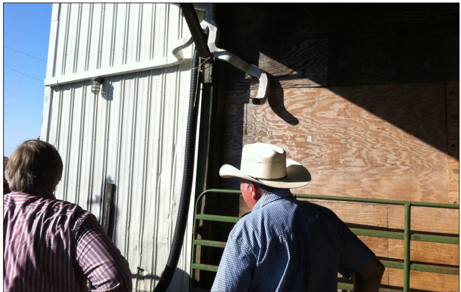
Figure 9. An example of a guttered confinement facility with a diversion for diluting manure pits.
