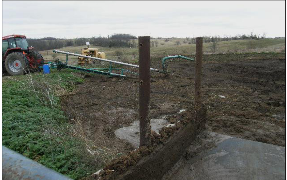
Figure 7. A poorly managed manure storage pond with inadequate freeboard space.
