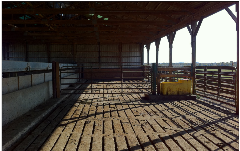
Figure 8. A confinement facility with a slatted floor and deep manure storage pit.
