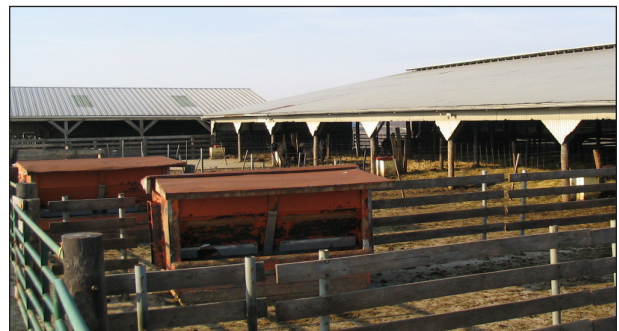
Figure 10. A partially-roofed backgrounding facility.
