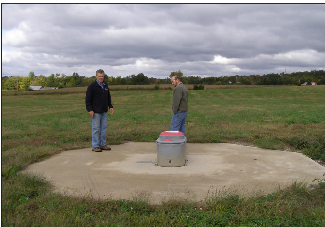
Figure 5. Octagonal concrete platforms provide a viable alternative to square concrete platforms. Photo by Steve Higgins.
