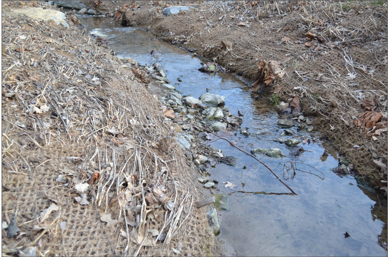
Figure 11. Erosion control blanket made of natural fibers.
