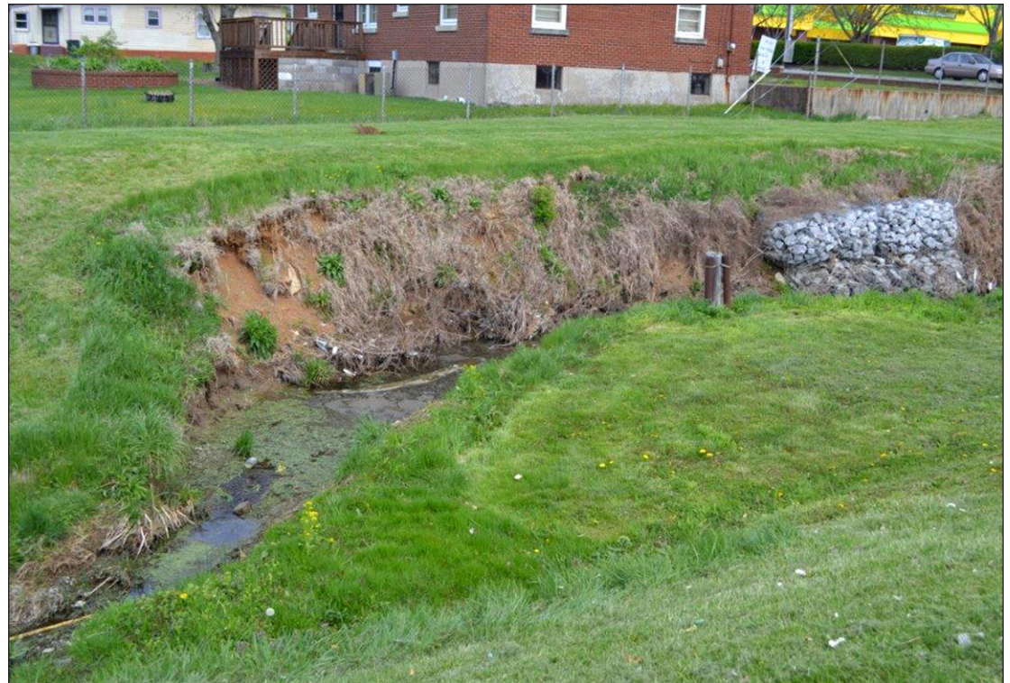
Figure 1. Stream exhibiting typical urban stream problems: grass mowed to the edge, eroded banks, and artificial structures (gabion baskets) used to reinforce streambanks.
