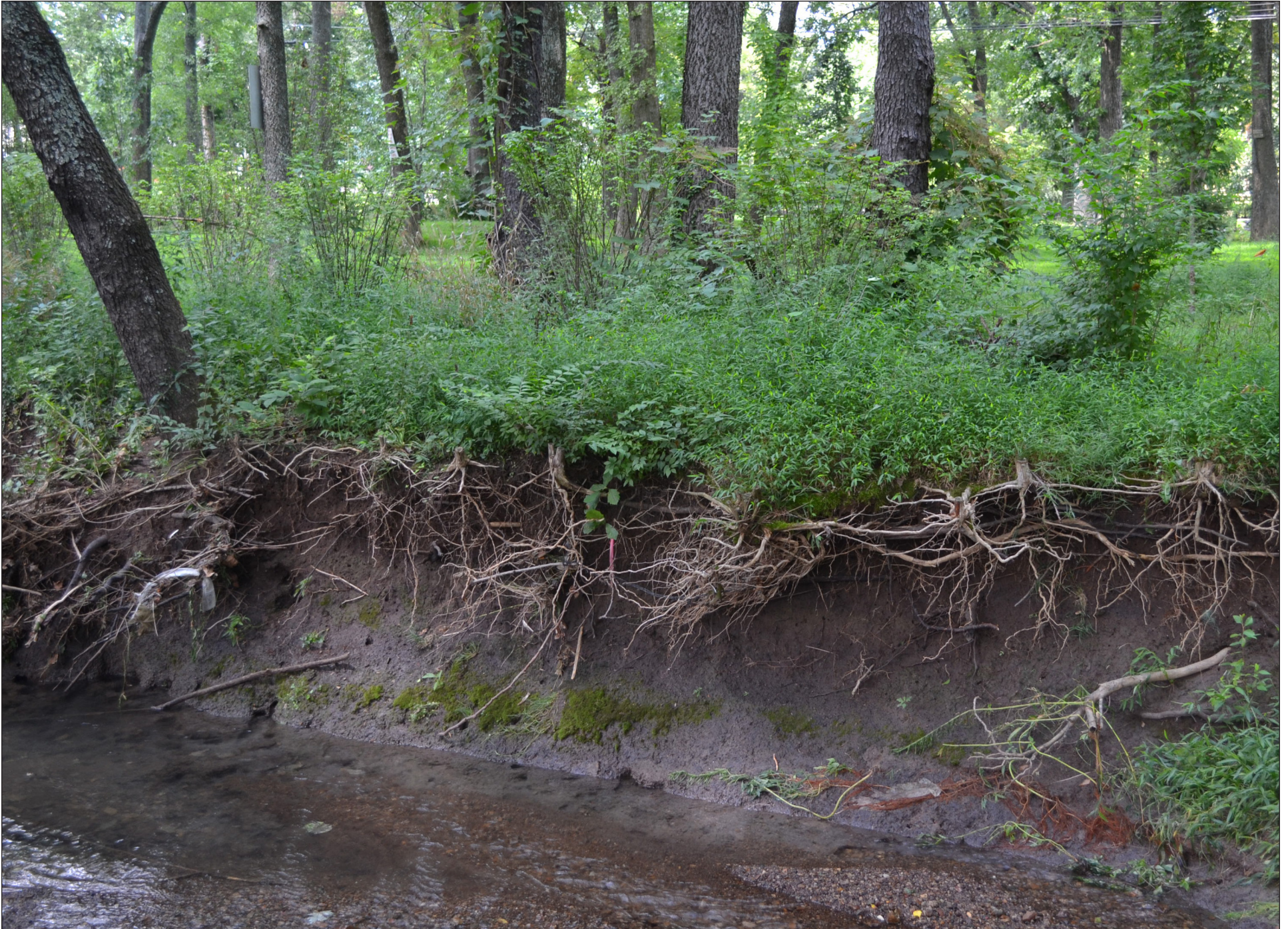
Figure 4. Eroding streambanks threaten private property and mature trees.
