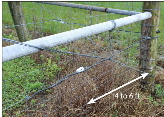
Figure 7. If the electrified offset wire is close to the existing fence at the start and end of runs, install the bull nose insulator 4 to 6 ft from the end post.
