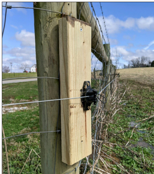
Figure 11. Gentle bends that pull toward the post can be made using heavy-duty wood post insulators. If the electrified offset wire is too close to the existing fence, then a treated 2" x 4" board can be mounted to the post.
