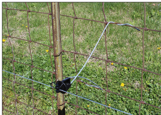
Figure 3. Wire-mount offsets are easy to install and remove. The straightforward design is ideal for older fences since the mounts are flexible and move with the fencing material, thereby reducing the chance of shorts.
