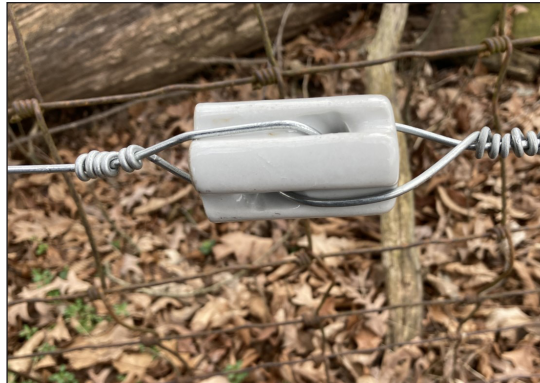
Figure 6. The beginning and ends of runs should be terminated using a bull nose insulator designed for high-tensile fencing.
