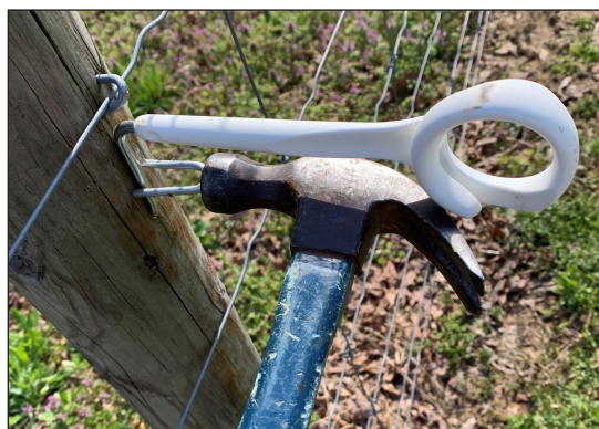
Figure 4. Offsets for wood posts are more rigid than wire mounts. The rigidity makes them a good choice to install at the beginning and end of runs where there will be additional pressure pushing back against them.
