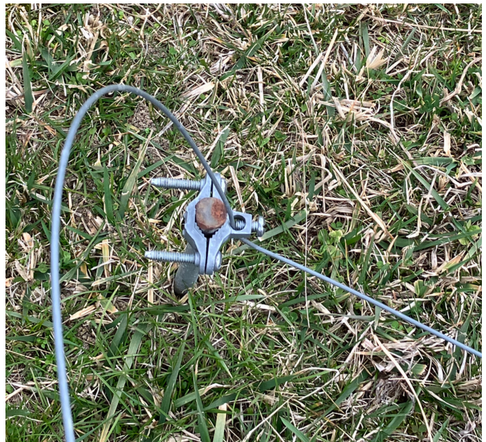
Figure 5. Ground rod clamps ensure a strong connection between the ground rod and the connector.
