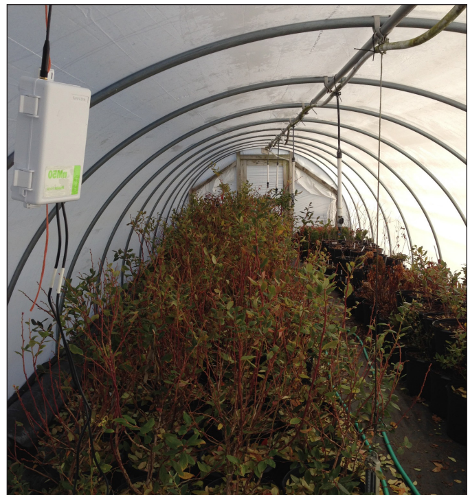
Figure 2. nM50 node in overwintering house to send media moisture sensor readings to office.
