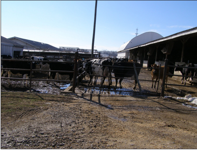
Figure 1. Over the years, gravel has been added to this driveway, increasing its height so it now drains into the production area.
