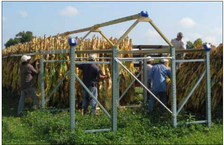
Figure 6. Hanging stick tobacco in a pallet rack structure.
