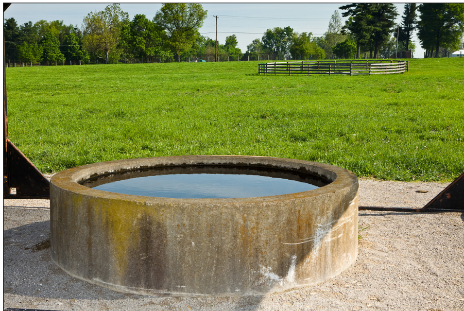
Figure 5. This tank is fed by the fenced developed spring in the background.
