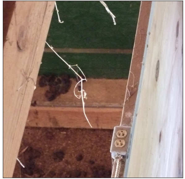
When hay is stored in the barn loft, pieces of hay may accumulate on the trusses and may fall inside the electric outlet, creating a spark and possible fire.
