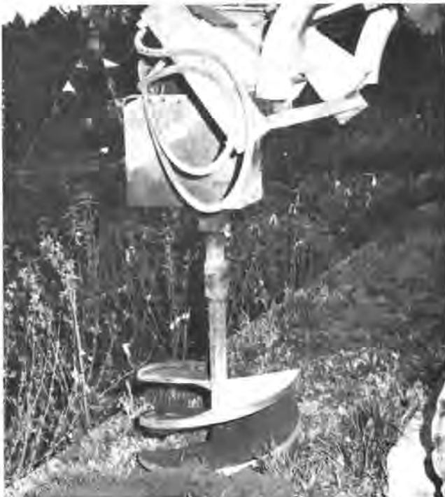
Figure 4.—Digging the planting hole with an auger.
